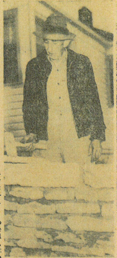
"UNCLE CHARLIE" ... builds fence
